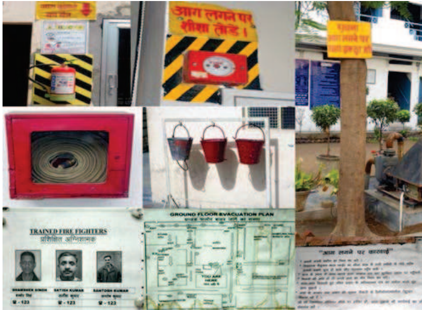
Plate 2 Fire safety Instruction & equipment
